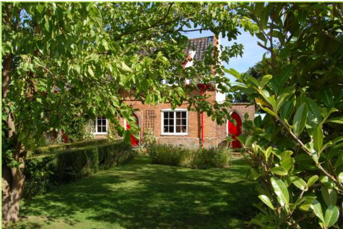
Fig 15, No. 21 Southwold Road
