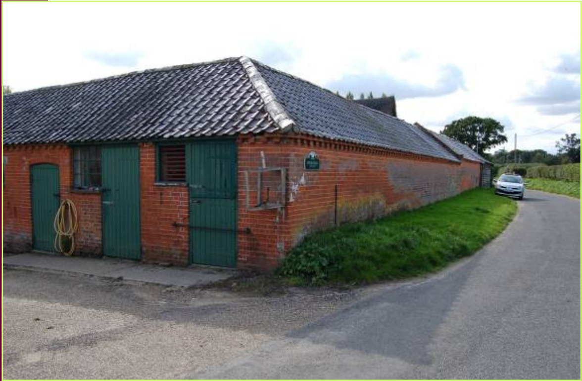
Fig 23, Farm buildings, Priory Farm, Priory Road
