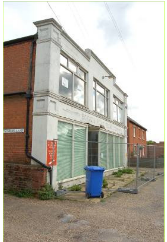
Fig 2, No 26 High Street, former Boggis electrical store
