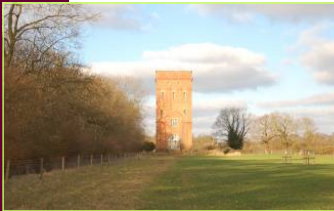
Fig 33, Water Tower, Benacre Park
