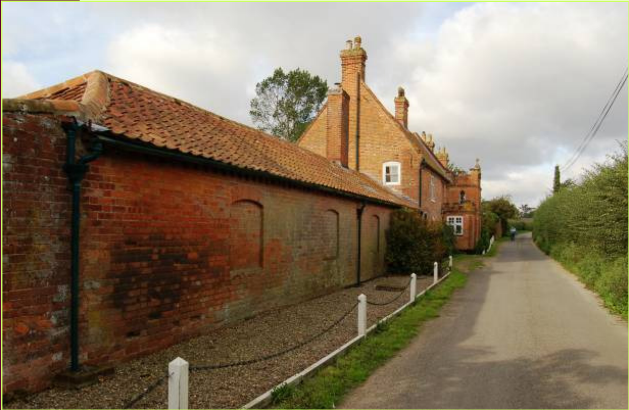
Fig 16, The Priory, Priory Road
