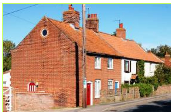
Fig 17, Nos. 6-14 Southwold Road
