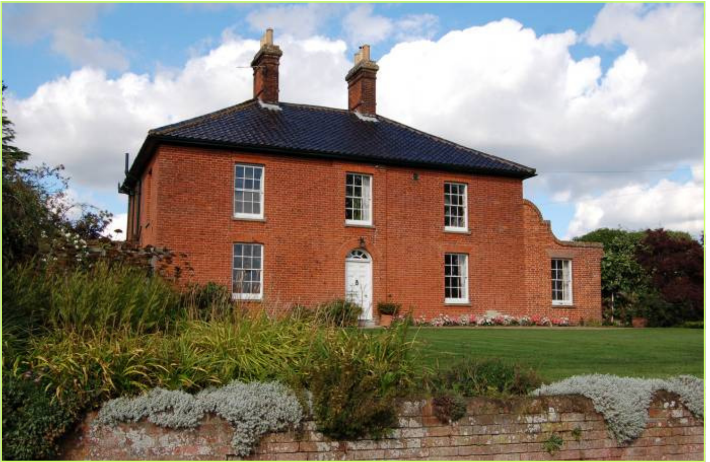
Fig 14, Priory Farmhouse, Priory Road
