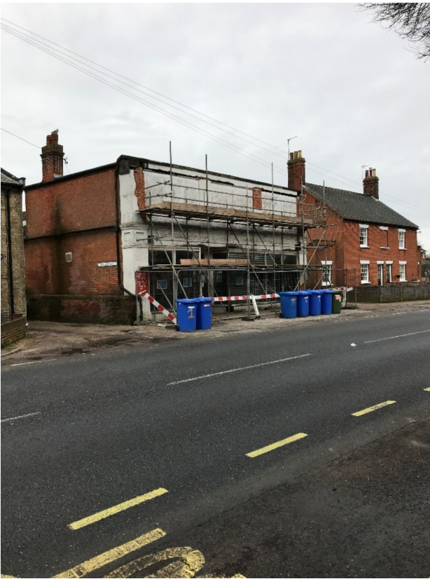
Photo 21.02.2020 - work on the front of the building.
