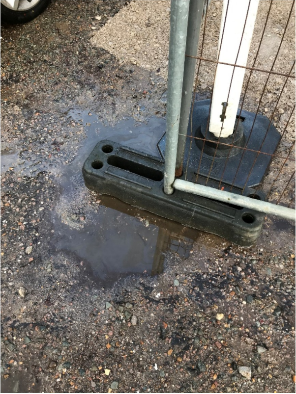
Photo 21.12.19 - at the foot of one of the fencing corners.
